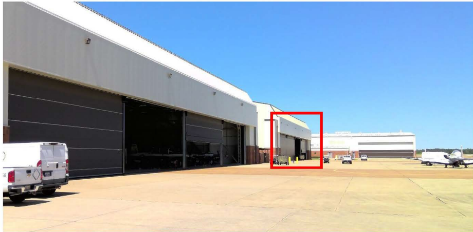
Figure 4. Image showing a recent example of vertical lift doors being used on existing DAF hangars (image provided by DAF). The color option on the right, noted in red, would be the approximate color of the doors that would be used on Building Nos. 452 and 454.
