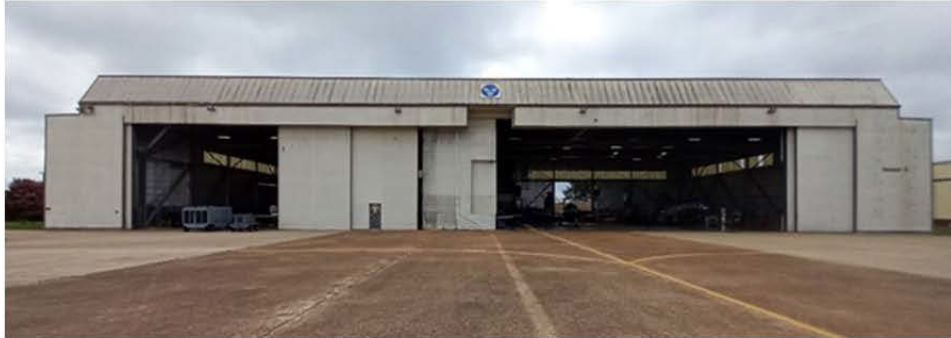
Figure 2. Image showing the current hangar doors and façade.
