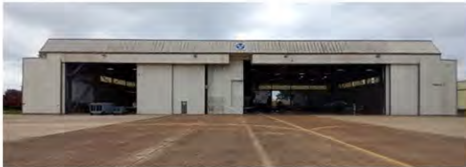
Figure 2. Image showing the current hangar doors and façade.
