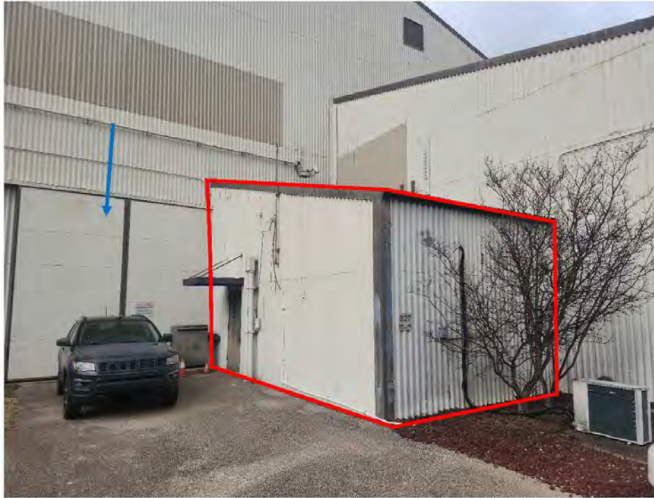
Figure 21. Detail showing the ca. 1980 addition on the rear elevation indicated in red, which partially covered an existing door indicated by the blue arrow.
