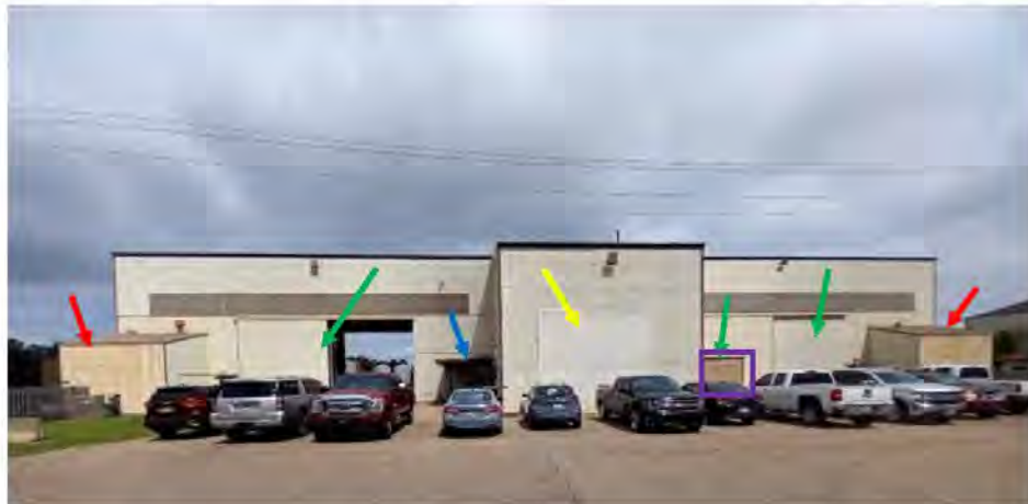
Figure 10. Image showing the current configuration of the southeast elevation. The additions indicated by the red arrows would be removed. The canopy indicated by the blue arrow would be replaced in-kind. The doors that would be removed are indicated by green arrows. The roll-top door noted in Figure 11 below is outlined in purple. The infilled nose dock is indicated by the yellow arrow.
