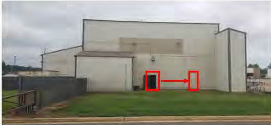
Figure 22. Image showing the current composition of the northeast elevation. The door indicated in red would be replaced with a new single-leaf steel door and shifted in location to allow for a small addition to the mechanical room.
